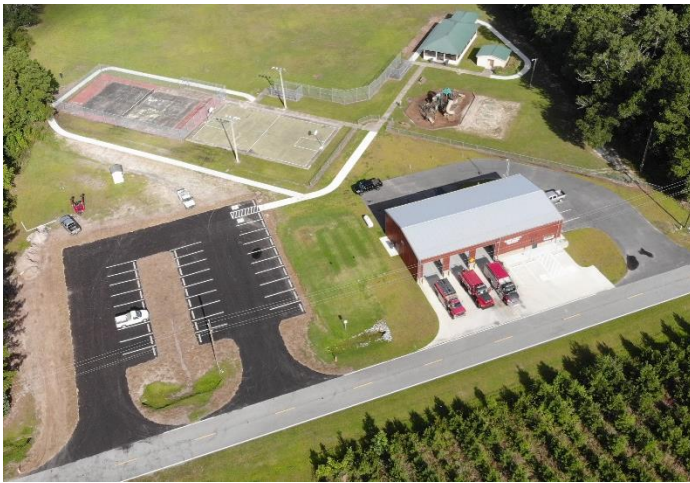
New Parking Lot (right), Firehouse 18 (left), and Mary B. Smart Park (back)
